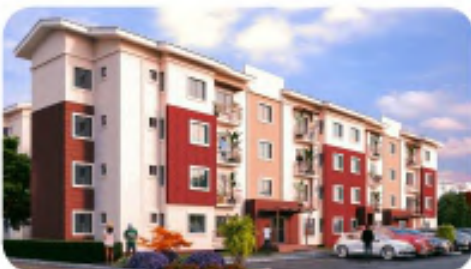
2 & 3 Bedroom block of flats in Fara Park II, KM 22, Lekki-Epe Expressway, Lagos
